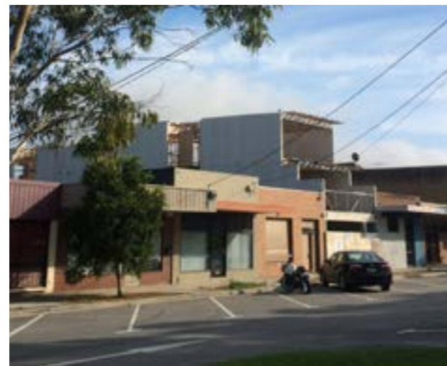
Lewellyn Place, Eumemmerring: Shop Top Housing under construction
