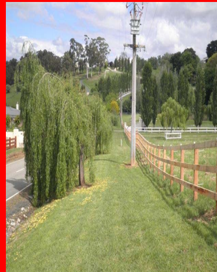
Figure 3 Unconstructed Road Side Trails
